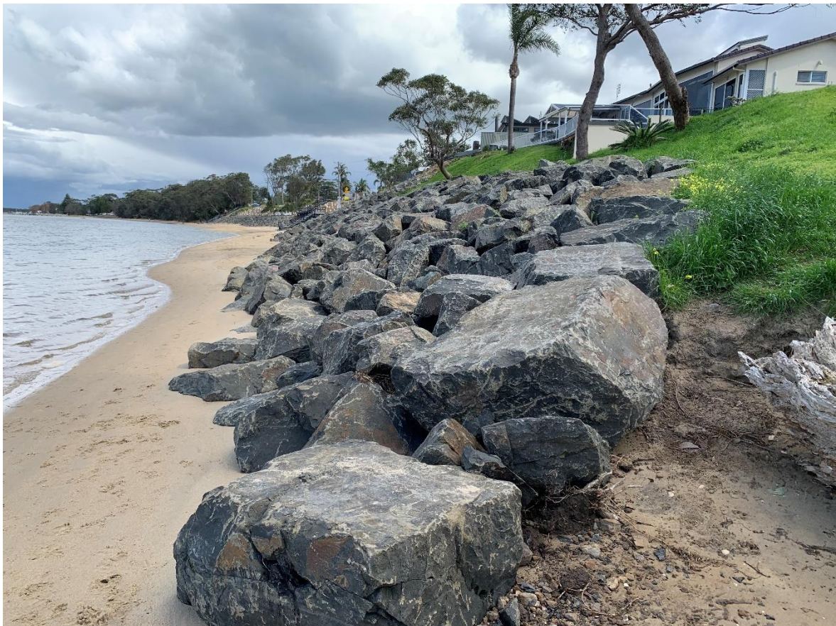
Figure 3.6 Eastern end section of rock revetment (Ch 680 - 720 m)
