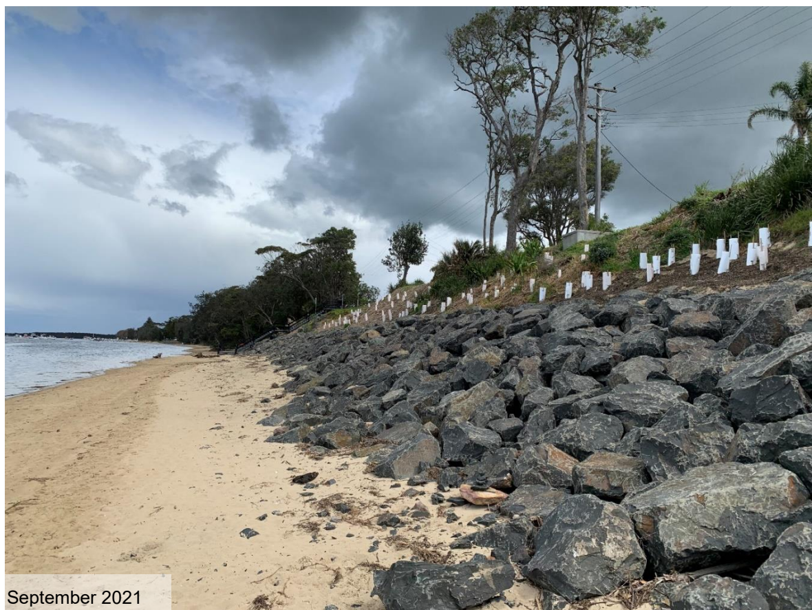
Figure 3.2 Western end of rock revetment, at Ch 550 m looking west
