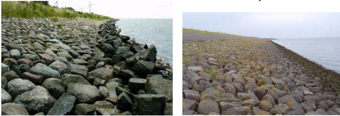
Figure 5.8 (L) Pitched rock slope with randomly dumped rock in front. (R) Pitched rock slope (Nurmohamed et al., 2007)
